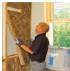
2. SWIP Batt between SWIP Studs
