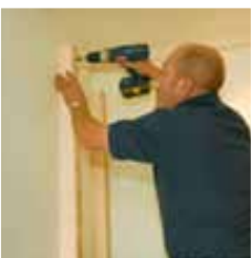
1. SWIP Studs fixed to wall
